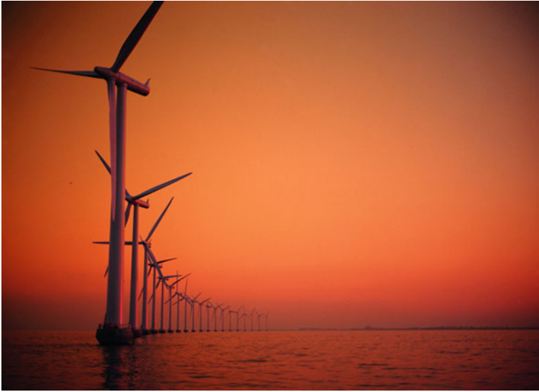
Fig. 5.30 An offshore wind farm at Middelgrunden near Copenhagen, Denmark. Each rotor blade is 36.8 m long. (Courtesy of LM Glasfiber, www.lmglasfiber.com )
