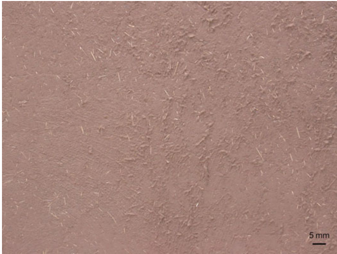
Fig. 1.1 Straw reinforced adobe wall in Taos pueblo in New Mexico, USA
